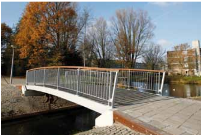
Bridge with plastic deck
